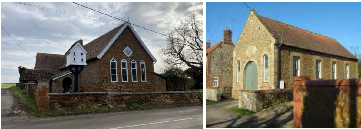
Figure 40-Old School (Y:1852) and former Methodist Chapel (Y:1865)
