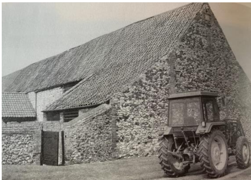
Picture of the large barn at Gedding's Farm dated 1630 within Susanna W Martins (1991) Historic Farm Buildings Book 4 .
