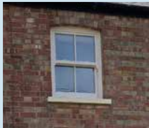
Sash window and details
