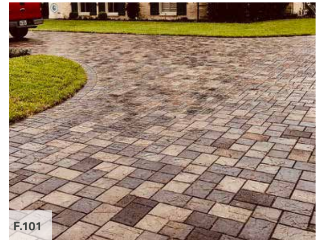
Figure 101: A good example of permeable paver (Source: https://www.paverconnection.com/testimonial/hedwig-village-permeable-driveway-and-patio-upgrade/ )
