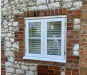
Casement window and red brick dressing
