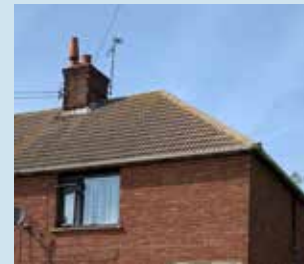
Hipped roof with concrete tiles
