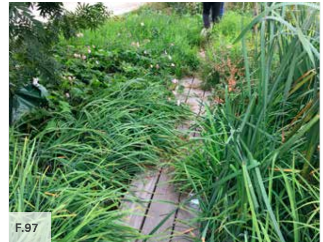
Figure 97: Examples of SuDS designed as a public amenity and fully integrated into the design of the public realm, Sweden
