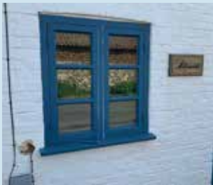
Casement window with painted timber
