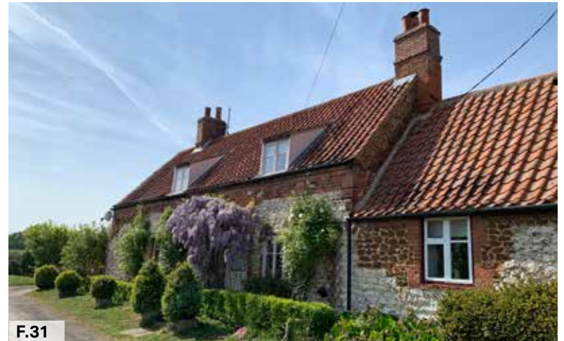
Figure 31: Terraced houses built with a mix of white clunch and carrstone and shed dormers on Chapel Lane
