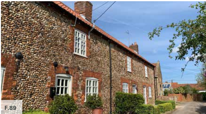
Figure 88: Mix of carrstone and red brick on wall and use of red brick as decoration around casement windows
