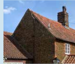
Gabled roof and red pantiles
